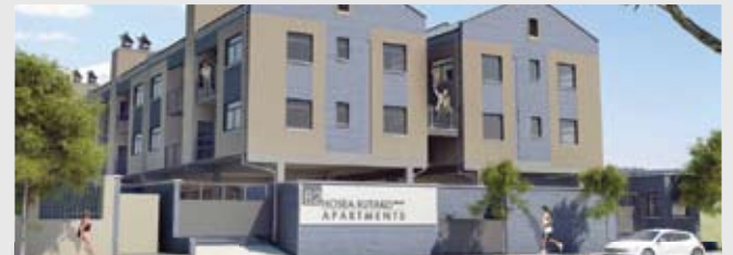
Hosea Kutako Apartments
