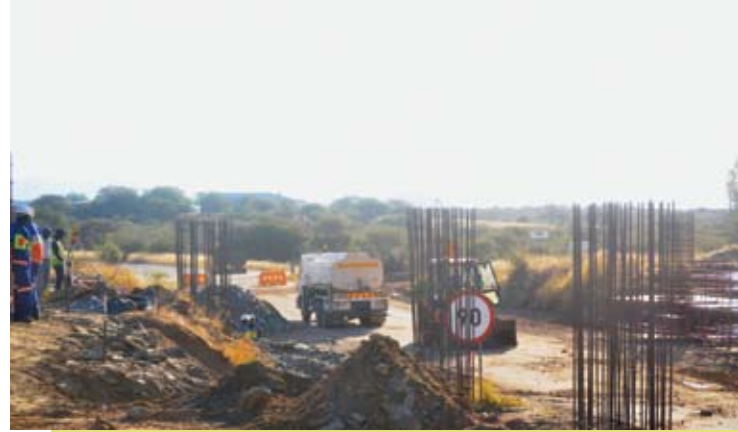
CONSTRUCTION BOOM: Construction activities have surged in 2014
