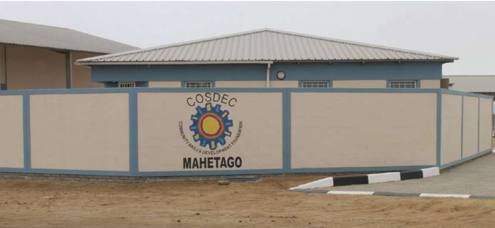
The brand new COSDEC facility at Swakopmund (Mahetago) built with financial assistance from the Millennium Challenge Corporation (MCC) through MCA Namibia.
