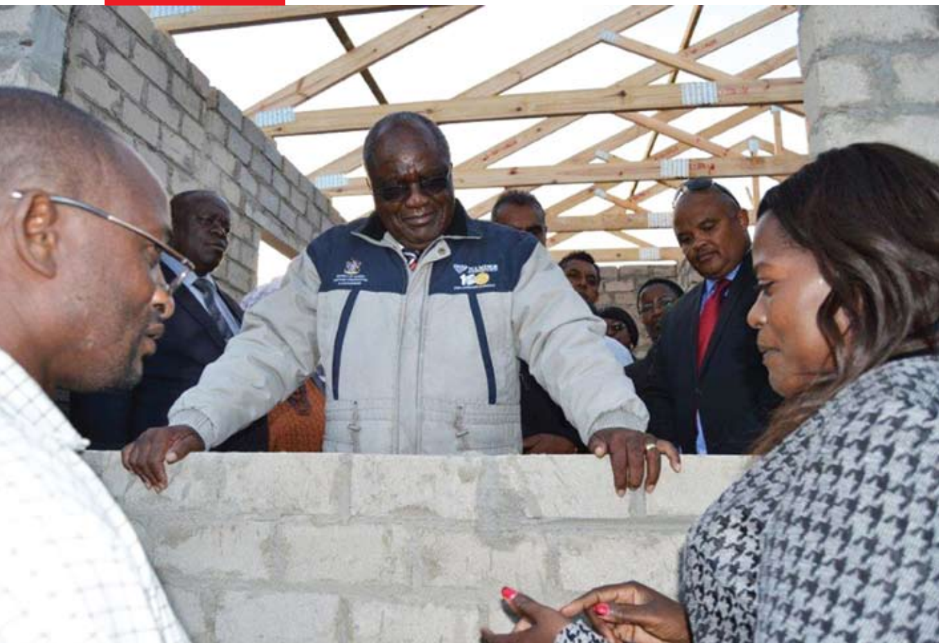
President Pohamba visits mass housing project at Walvis Bay
