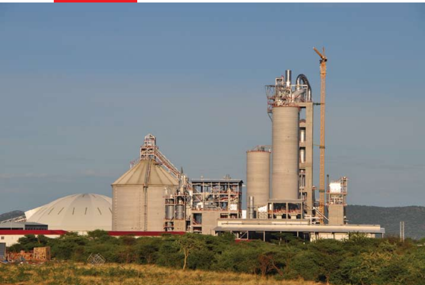
SETTING STANDARDS: The Ohorongo Cement plant just outside Otavi.
